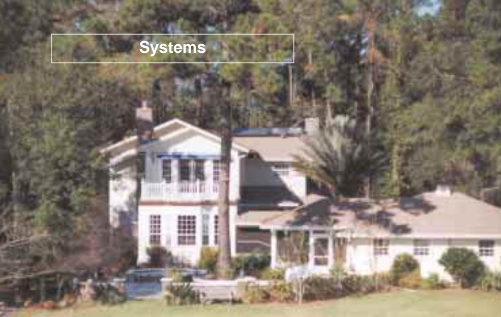
Above: The Ford house has a solar hot water system with panels on the roof.
